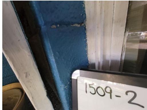
1509-2 Caulk/White (2% Chrysotile) Typical Exterior Windows
