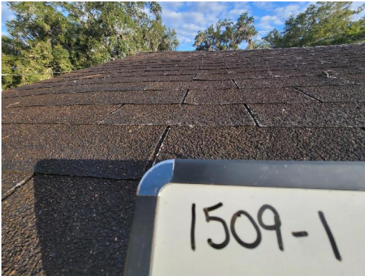
1509-1 Asphalt Shingle Typical Exterior Roof
