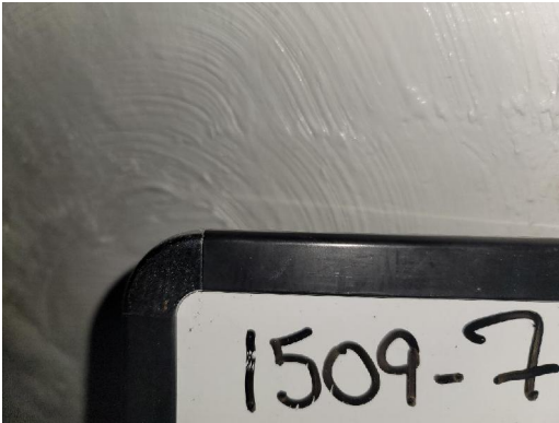
1509-7 Plasterboard (Shower) Interior Bathroom
