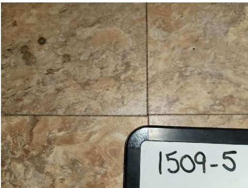
1509-5 2'x2' Floor Tile/Adhesive Interior Southwest Bedroom
